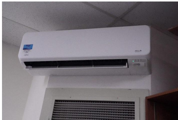
Figure 2 Wall-Mounted Mini-Split System
