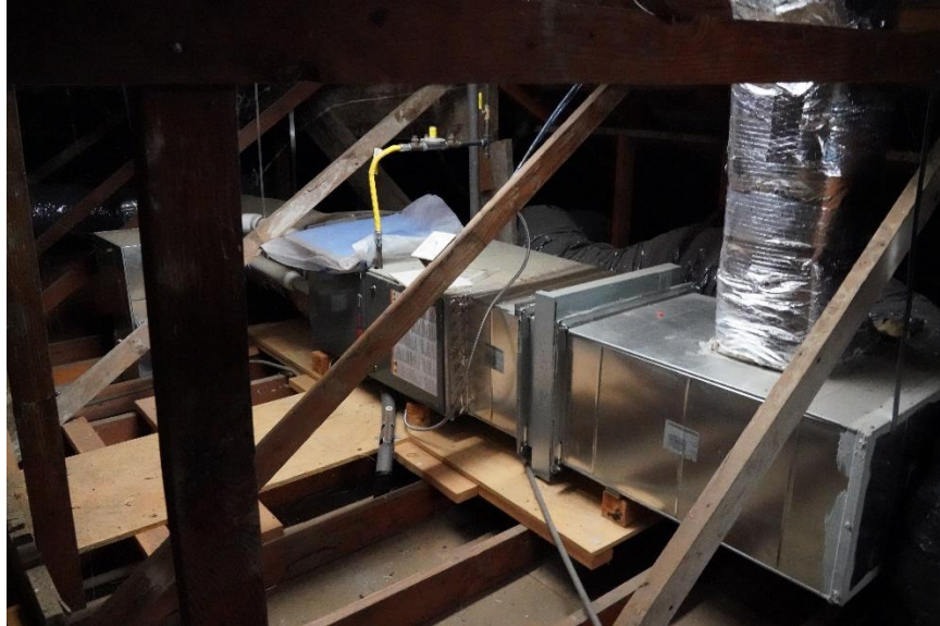
Figure 3 Trane XR95 gas-pack air handling unit
